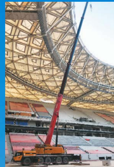
Al Janoub Stadium, Qatar
