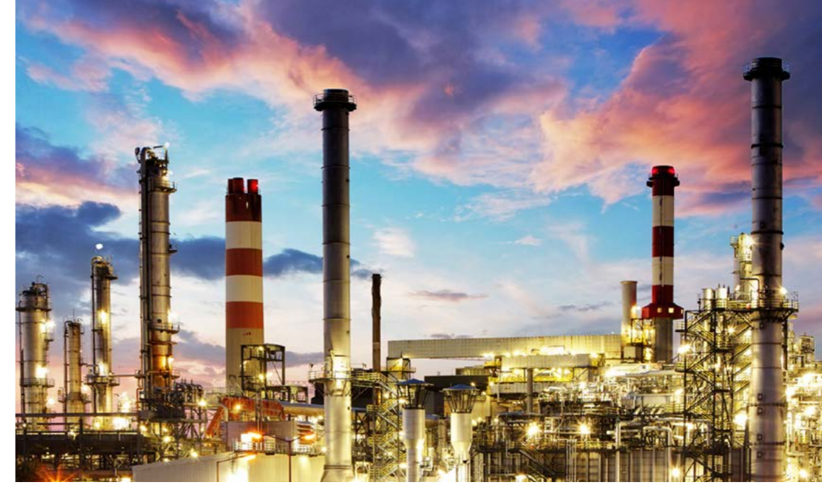
Dangote Refinery, Nigeria
