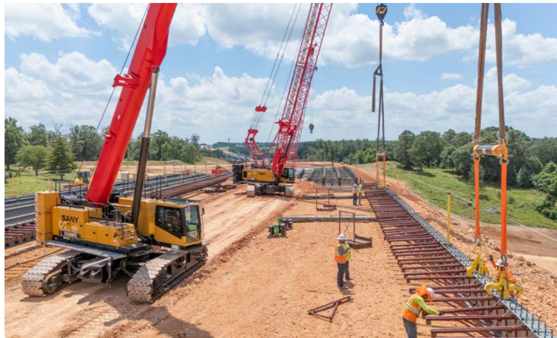
Bridge Construction, Arkansas, USA
